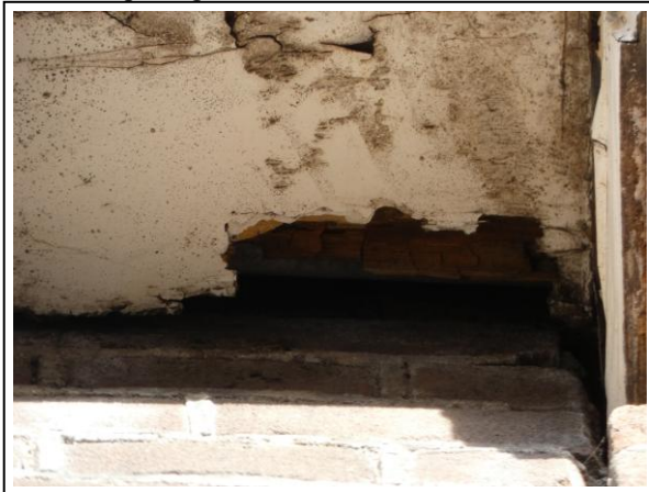
Foto 5 opening in dakrand
