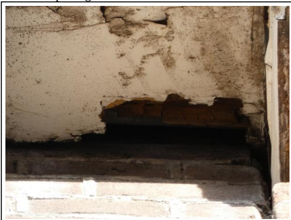
Foto 5 opening in dakrand
